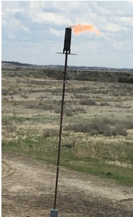
Figure 5: Existing Flare That Was Replaced
