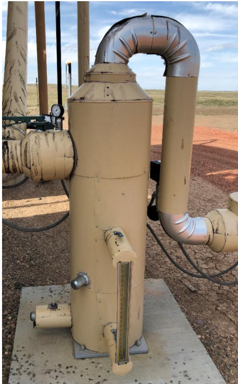
Figure 4: Vertical Knockout Vessel with Pocketed Discharge Line
